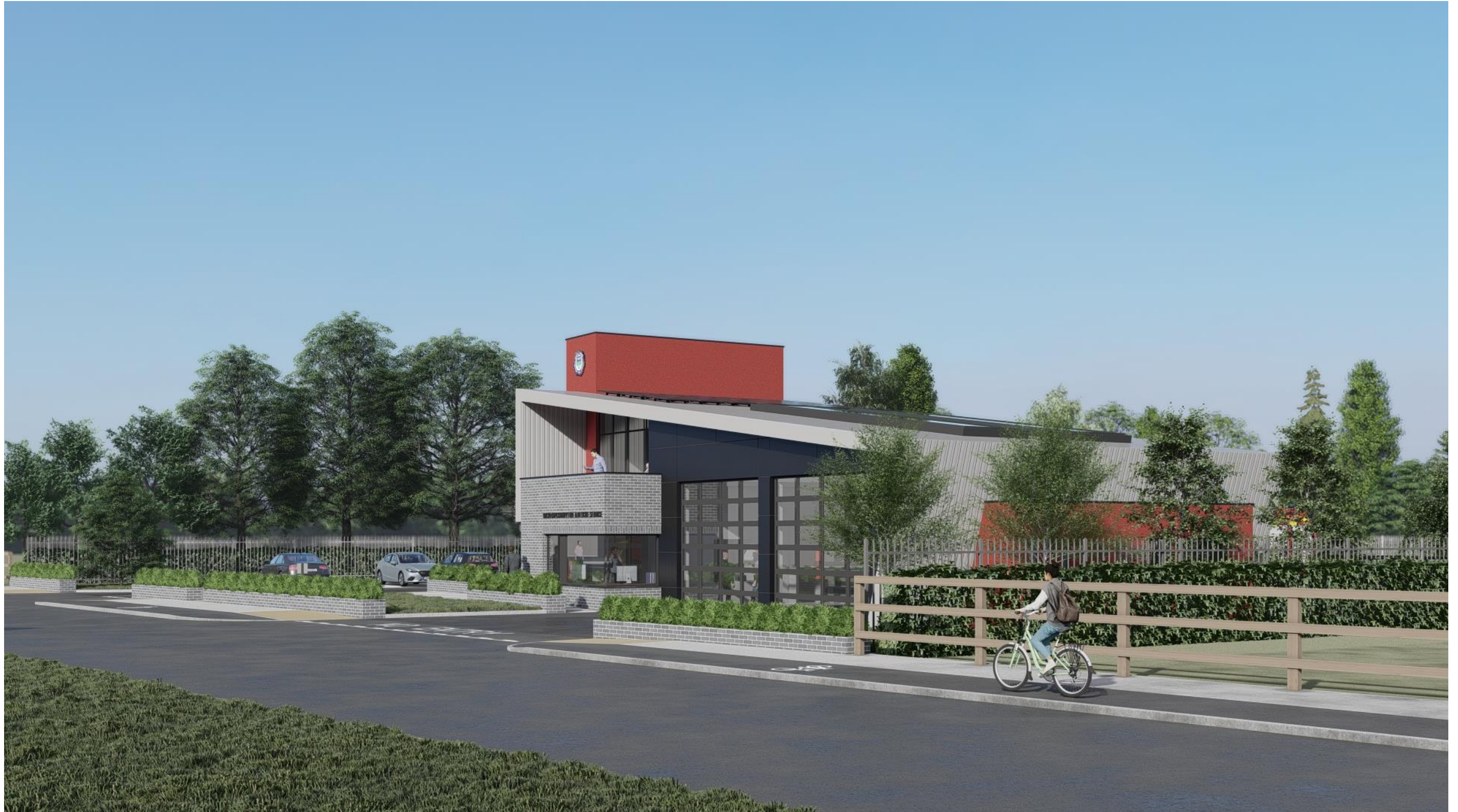
Figure 12: Overall View from Main Road
